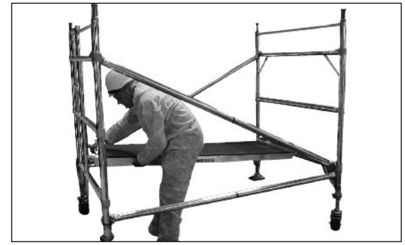
5 Fit plain platform on appropriate rung of frame. See tower kit guide for illustration. This will indicate which rung to fit trapdoor platform depending on final tower height.
