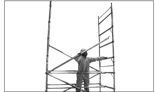
10 Klik in diagonal braces to continue in a regular pattern. Double width towers always have diagonal braces either side of the tower opposing each other as illustrated.
