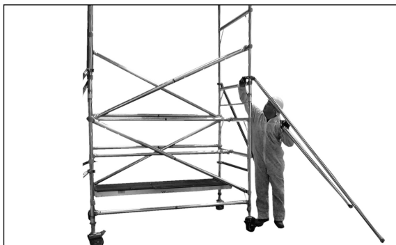
11 Secure stabilisers as soon as possible to increase tower stability. Check tower kit list to ensure the correct stabilisers are fitted.
