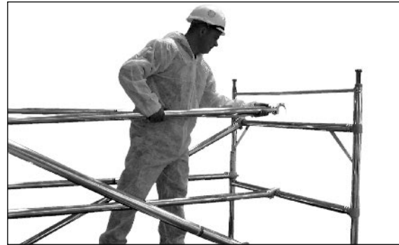
7 Fit four handrail braces, two on outside and two on mid rung of frame as shown, on lower levels these may not be required.
