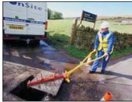
Slide the cover back on the Ezi-lift rollers
