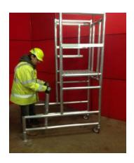
5) CLIP UPPER BRACE OF LADDER ABOVE RINGS ON VERTICALS WITH ASSEM-BLED HOOKS AT TOP
