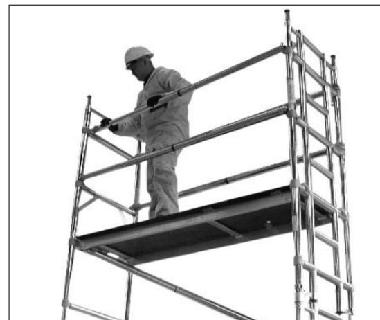
14 Dismantling is the reverse except when dismantling the handrail braces. Unclip the far end hooks and then from the sitting position through the trapdoor (3T) remove the handrails. Do not remove the handrails whilst standing on the platform, this would leave you at risk.
