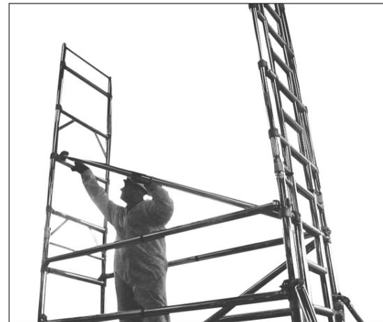
10 Klik in diagonal braces to continue in a regular pattern from rung to rung except when interrupted by an intermediate trapdoor platform.
