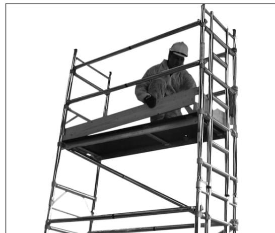
13 Fit toeboards when handrails and mid rails have been correctly fitted. For intermediate work, platforms, handrails, mid rails and toeboards must be fitted.
