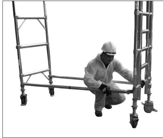
3 Klik in two horizontal braces to vertical member of the frame, as low down as possible.
