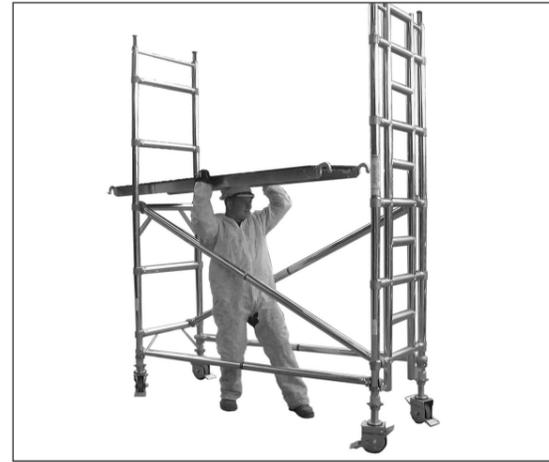
5 Fit trapdoor platform on appropriate rung, see tower illustration for guide. This will indicate which rung to fit trapdoor platform depending on final height.
