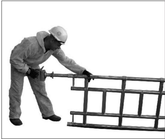
1 Insert two adjustable legs and castors into frame.
