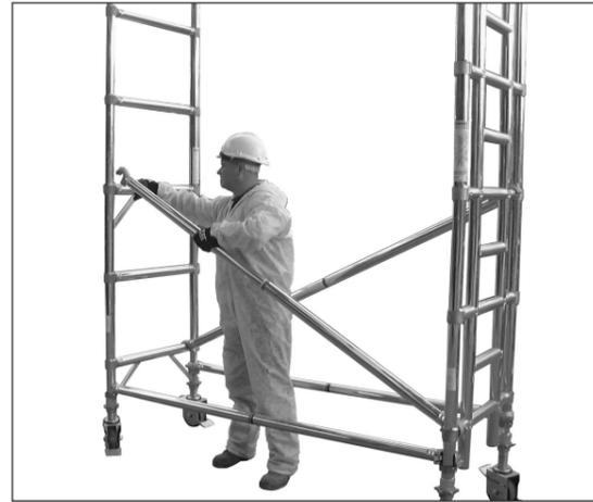
4 Klik in diagonal braces, starting at the bottom rung. Single width towers have 2 braces at the base and singular thereafter. Braces should be in a continuous pattern from rung to rung except when interrupted by an intermediate platform.
