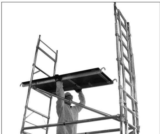
11 Fit trapdoor platform on appropriate rung. See tower illustration for guide.
