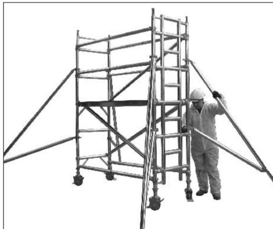
7 Lock castors and level tower. Secure stabilizers as soon as possible to increase tower stability. Maximum tower height is 8m. For heights greater than this, towers should be tied in to an adjacent building or structure.
