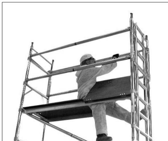
12 From the sitting position through the trapdoor (3T) fit four handrail and mid rail braces to the vertical members.
