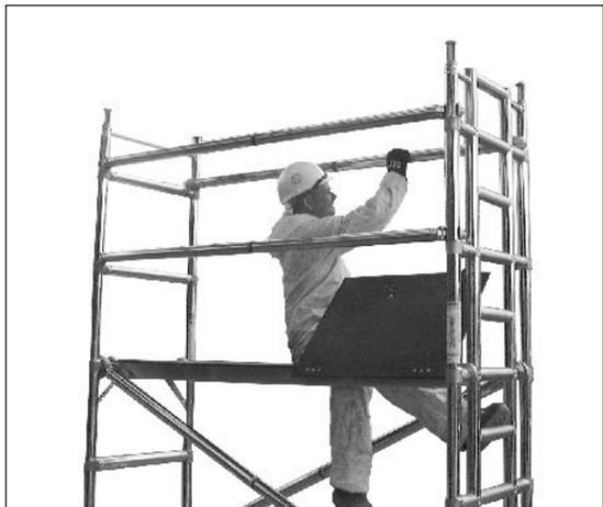
6 From the sitting position through the trapdoor (3T) fit four handrail and mid rail braces to the vertical member as shown.
