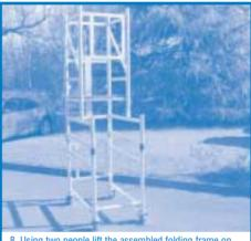
8. Using two people lift the assembled folding frame on top of the booster unit locating the uprights of the folding unit into the cups on top of the booster unit. Ensure all of the spring loaded pins in the cups are engaged into the holes in the frame.
