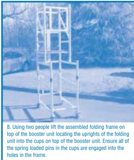
8. Using two people lift the assembled folding frame on top of the booster unit locating the uprights of the folding unit into the cups on top of the booster unit. Ensure all of the spring loaded pins in the cups are engaged into the holes in the frame.
