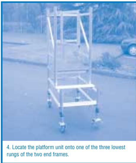
4. Locate the platform unit onto one of the three lowest rungs of the two end frames.
