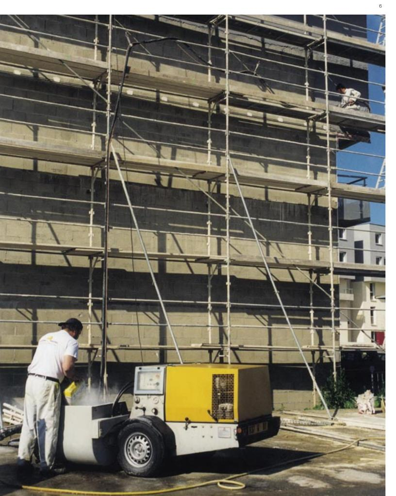
The SP 11 can also be operated by means of remote control from the spray gun so you do not have to depend on the machine operator.
