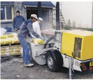
But that is by no means all! This SP 11 DMR has a lift mixer with powerful hydraulics to carry out the job.
