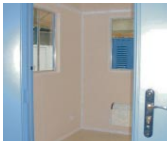
Entry to the unit is via new easy to use engineered doors. These doors are very strong but easy to operate. Each door is keyed separately to allow the client to decide on access to each area. This proves useful with a unit offering toilet, canteen, and office areas as it makes it possible to restrict access to certain sections.
