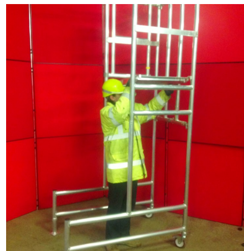
2) FIT PLATFORM AT CORRECT HEIGHT
