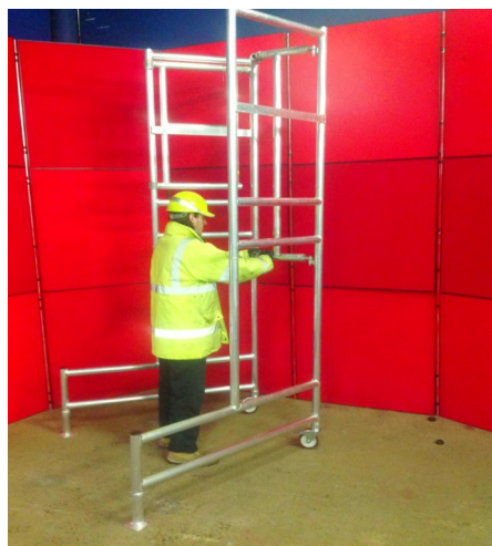
1) OPEN FRAME AND LOCK MECHANISM
